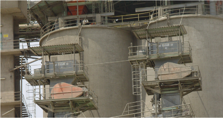
Figure 4: bucket elevators with the CFS's on top
