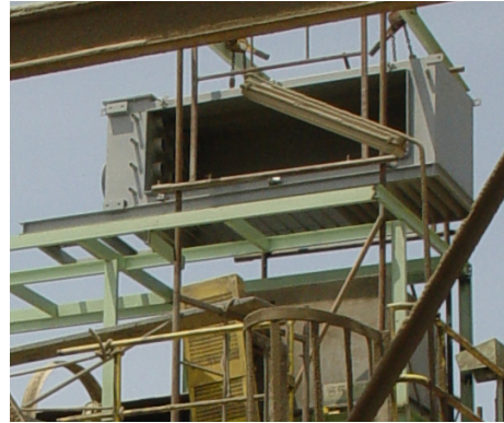
Figure 5: CFS dust collector over conveyor belt underneath clinker silo with overhead restrictions
