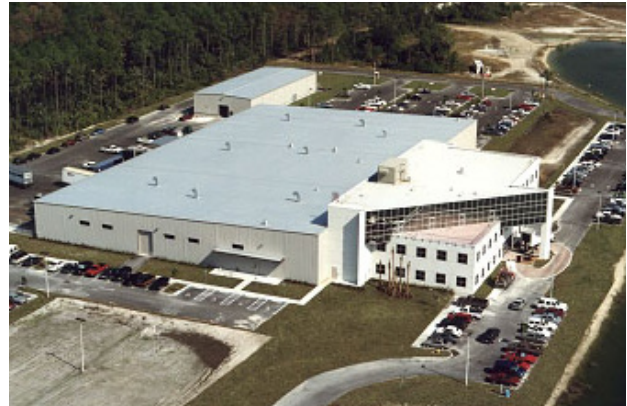
Parker Aerospace, Fluid Systems Division facility in Naples, Florida.
