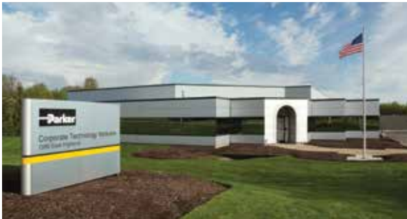
Parker's corporate technology ventures facility, Macedonia, Ohio.
