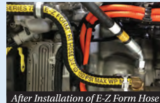
After Installation of E-Z Form Hose
