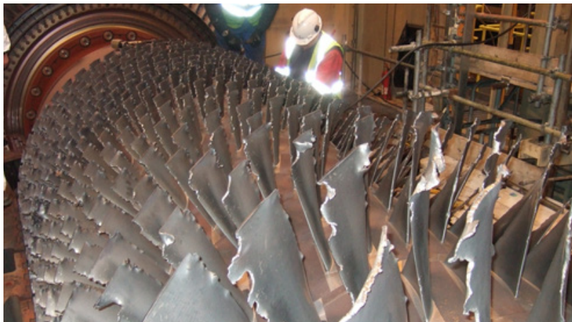
Fig. 5. Inadequate GT air intake filtration - corrosion pitting in this case led to crack propagation and ultimately compressor blade liberation.
