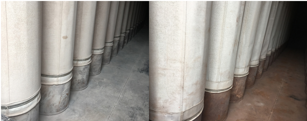
Thimbles and adjustable clamps leave room for error. See the correct installation location on the thimble (left) and incorrect installation point (right) that can quickly lead to loose, damaged or detached bags. Snapbands eliminate this user error.
